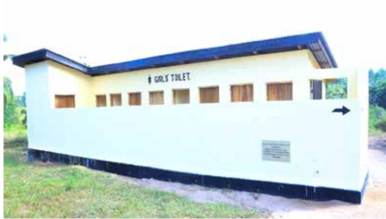
Figure 2: Girls' toilet constructed by HakiElimu at Dundani Sec. School, Mkuranga District
