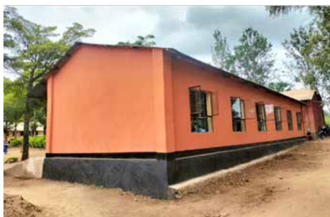
Figure 1: Classrooms constructed by So They Can in Mbulu District, Manyara.
